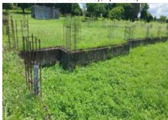
Plate No. 2.3-4: Foundation Part for the Construction of Phase II Building.
