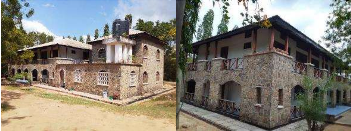
Plate 2.2: Hostels to be rehabilitated
